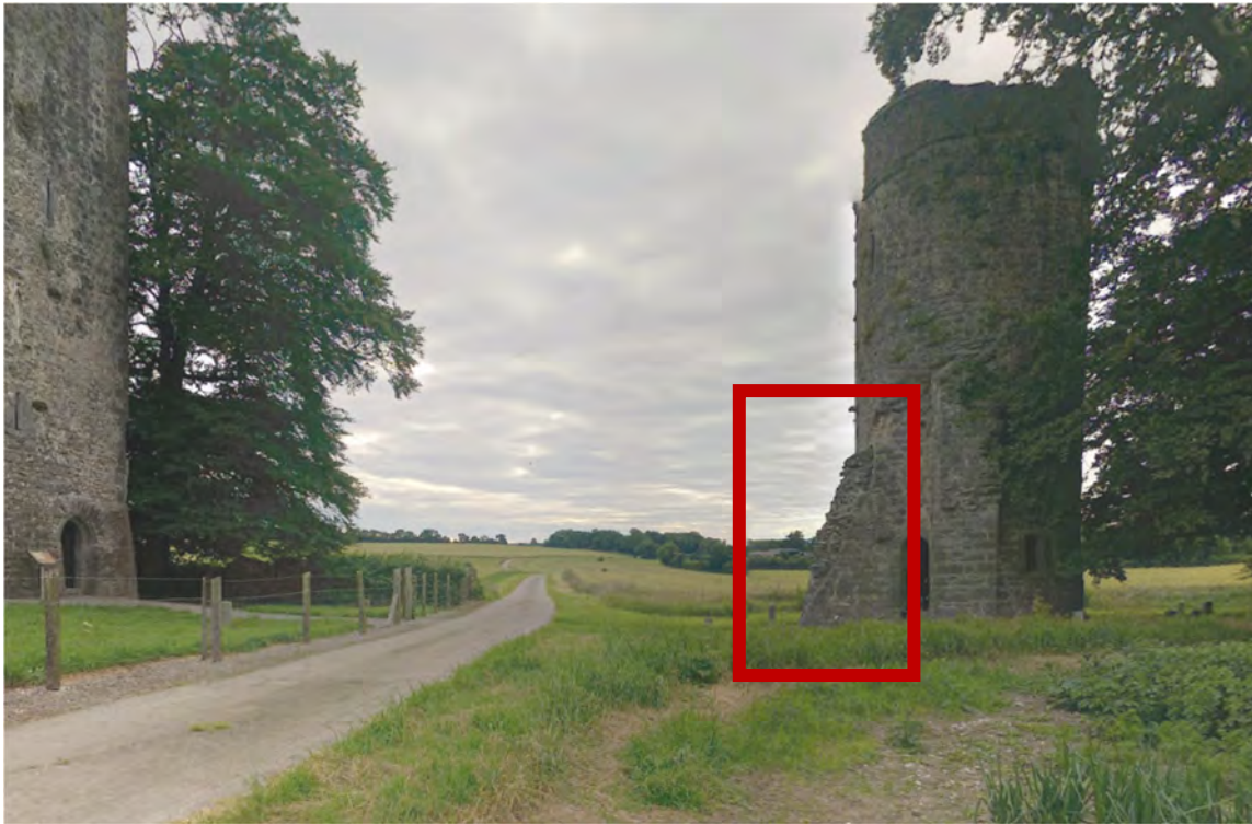
83- Burnchurch Castle Turret with Remnants of Historic Bawn (outlined in red) Source: Google Maps July 2016
