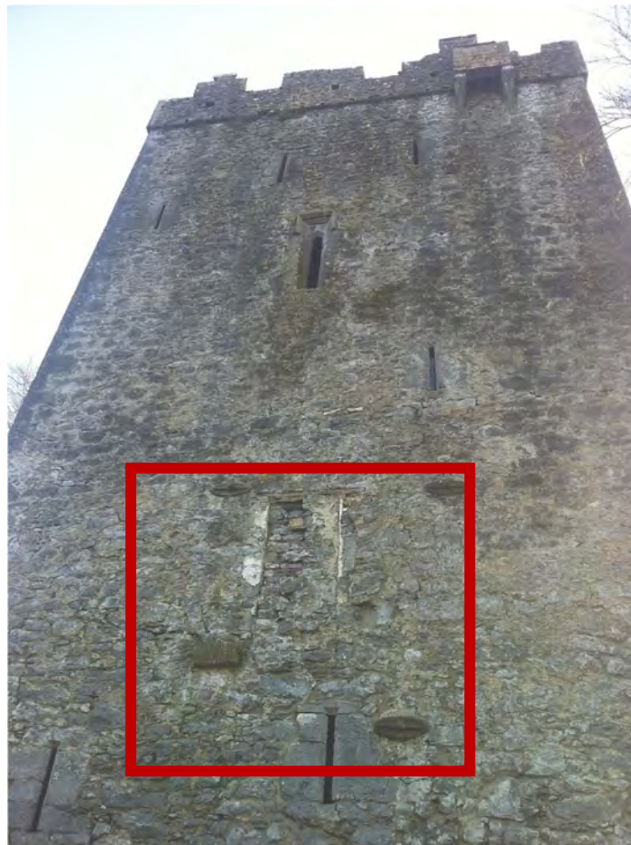
62- Extension Evidence on Northern Façade Corbels and Filled in Door (outlined in red) Source: Wikipedia 2024
