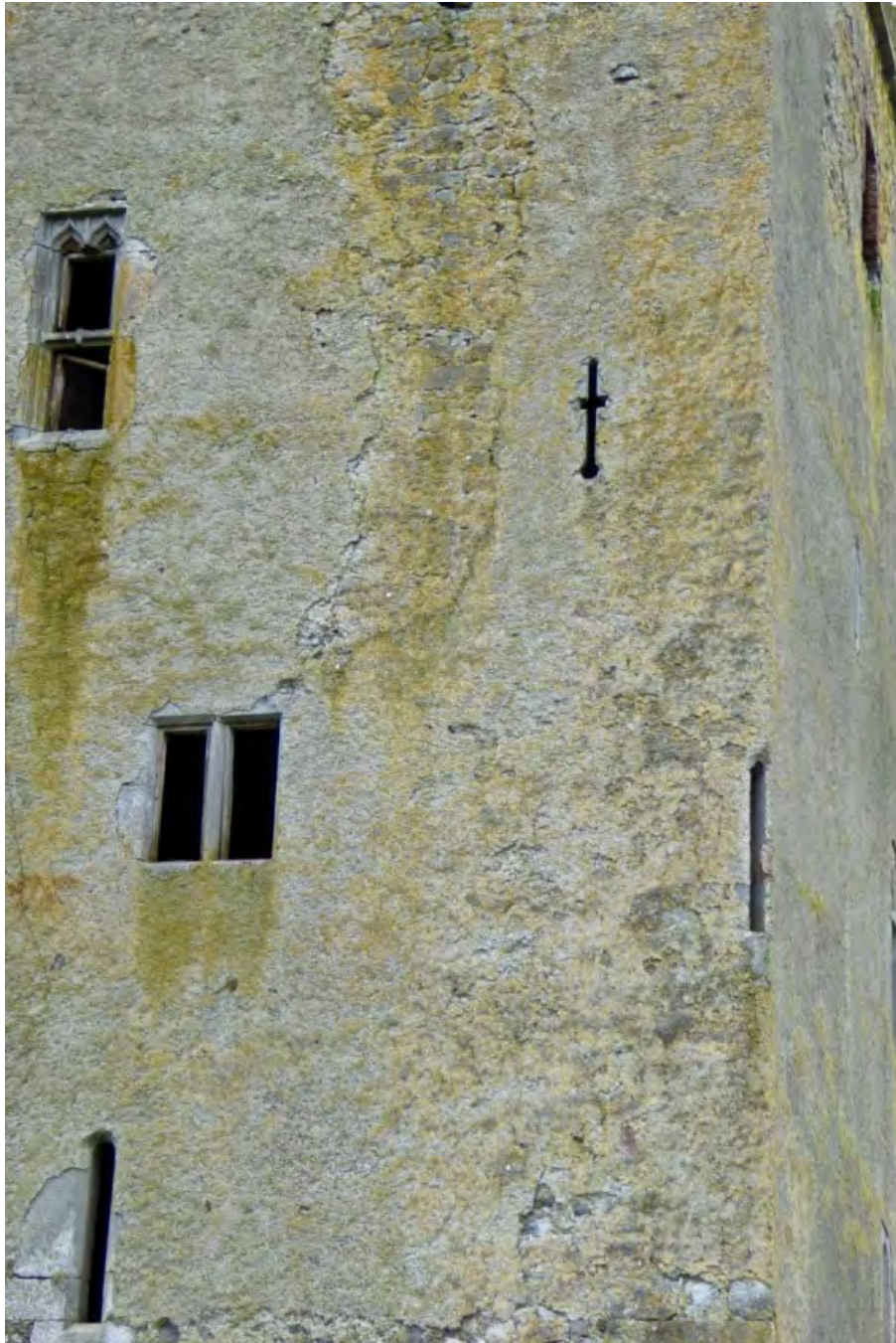
40- Arrow Loops or Arrowslits Source: Roaring Water Journal 2017
