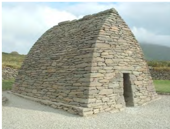
13- Preserved Stone Church circa. early 12th century at Gallerus, Dingle, Ireland Source: OPW, Ireland
